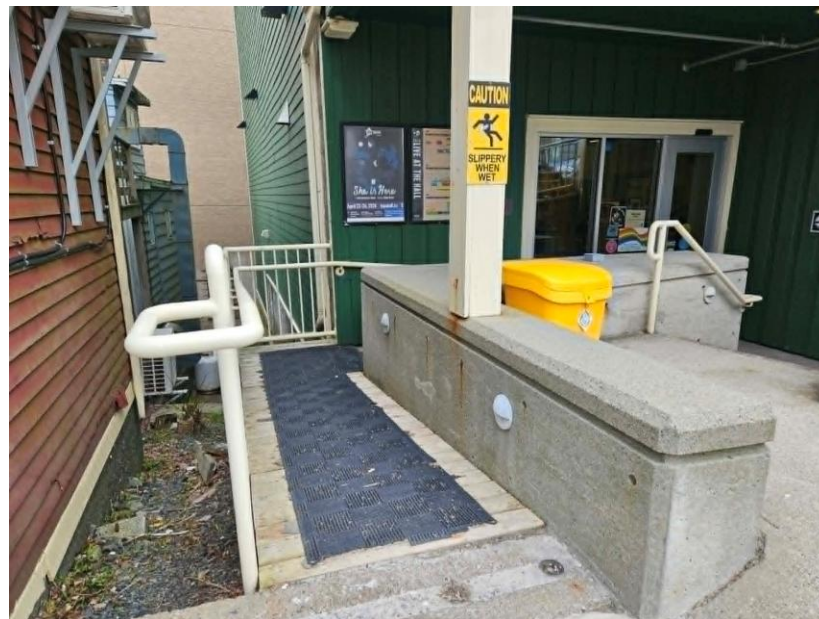
This is the ramp leading to the main door.
