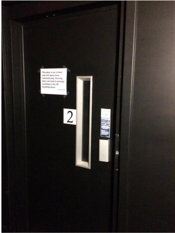
This is the door to the lift on the second floor.
